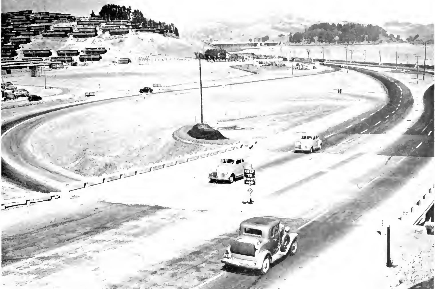
View of Waldo grade separation of U. S. 101 and Marin City road. Bridge structure carries 5-lane divided highway
